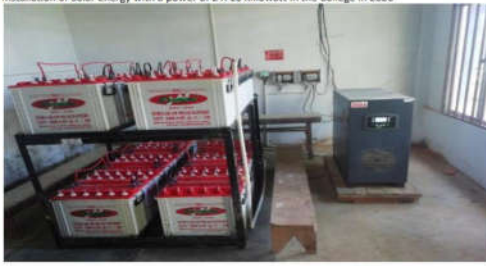
Installation of Solar Energy with a power of 2 X 10 Kilowatt in the College in 2020
